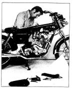
can use a spark boost. K-Mart coils or the new Andrews coils will give a useful energy increase; the bike will start easier, respond to the throttle cleanly and generally be more pleasant to ride. Pay close attention to the condition of the advance mechanism. When worn, the timing will vary and the bike may not want to idle. Keep it lubricat-
